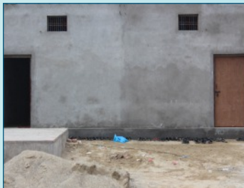
Work near to completion
