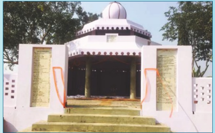
Project after completion
