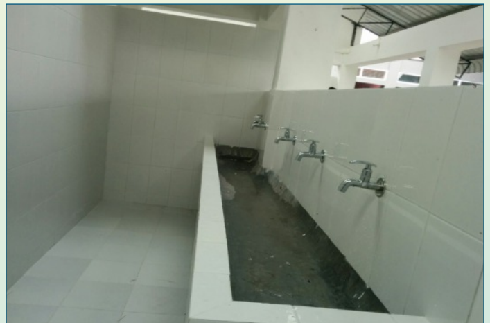
Completion of work
